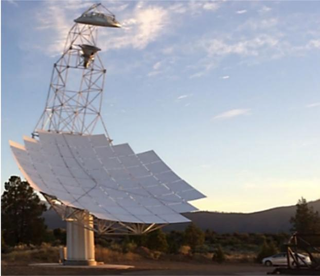
**Fig. 1** Segmented 13-m-diameter communication antenna dish with 60 thermoformed precision panels
